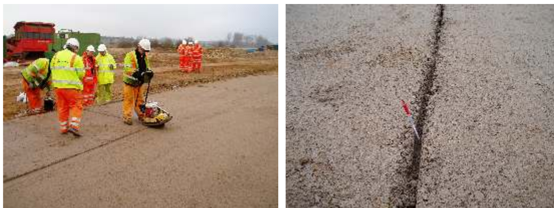
Figure 9: Induced cracking being carried out on a HBM subbase layer containing quarry fines
