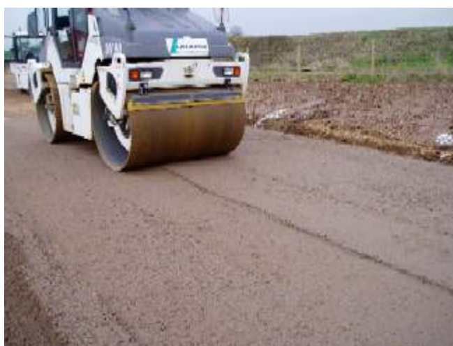
Figure 1: A HBM being compacted into a pavement foundation layer
