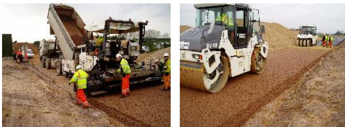
Figure 8: HBM being laid and compacted using conventional plant
